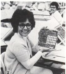
Control Store Board (UCS) installed in the microprocessor section of the computer as a permanent part of its processor instructions. Up to 2,056 words of RAM can be stored on a single UCS board.
